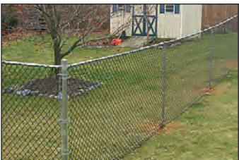
Chain Link Fence
